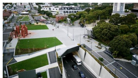
Figure 3: The fixed ramp to main entrance is located above Arras Tunnel
